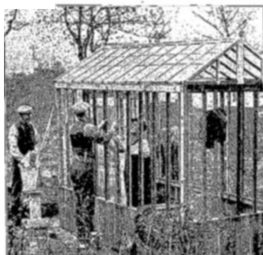
Figure 29. Men at the Warriston site constructing a greenhouse from old photographic plates. ( The Scotsman January 1935)
