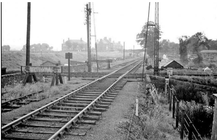
Figure 31. An undated photograph from the railway with the main site in the top right hand corner with the cottage just visible. ( EdinPhoto , www.edinphoto.org.uk )
